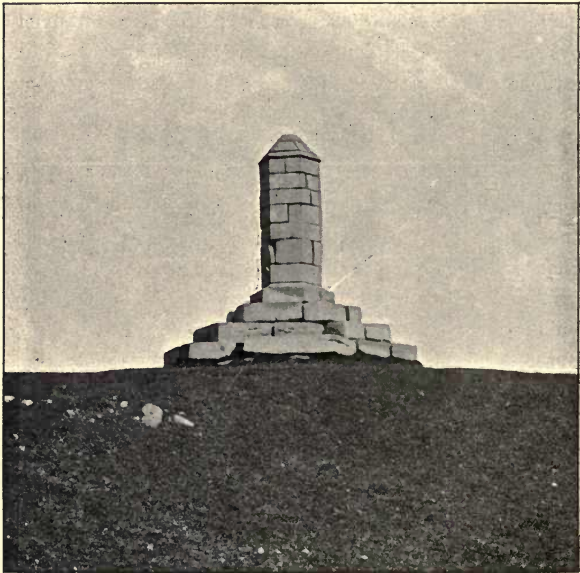
Monument of hewn, unmortared stones, on a mound close to the sea, New Quay, co. Clare.
